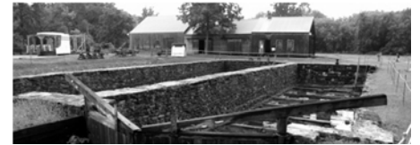
Dry docks at Chittenango Landing
